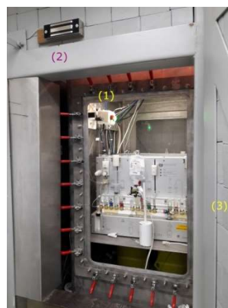
Figure 1. FDG cell: radiation monitor (1), magnetic door lock (2) and cell door (3)
